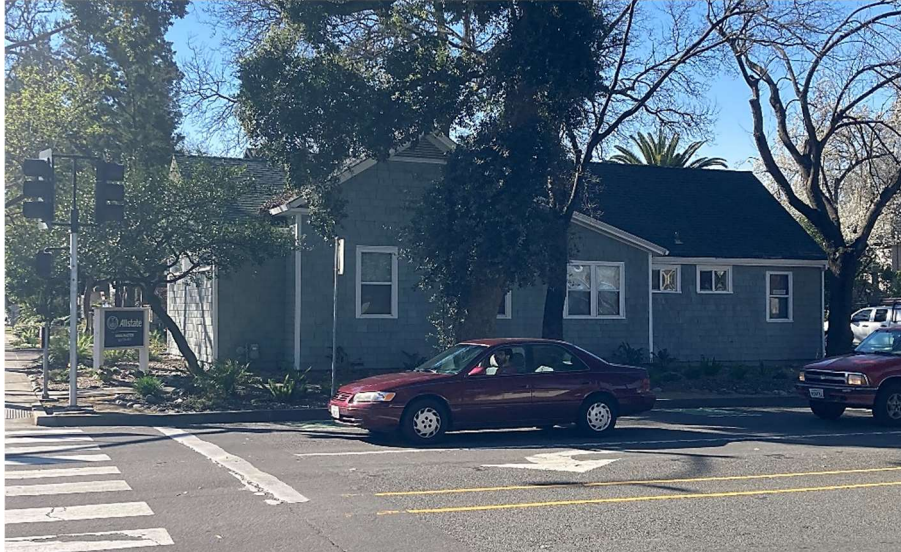
North façade, view facing south. Source: ESA, 2024.
