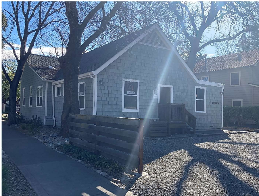
West façade, view facing southeast. Source: ESA, 2024.
